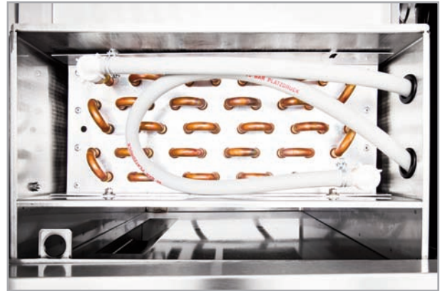
C20 Heat Exchanger
